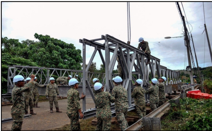
Picture 2: Military Personnel From 91 Support Regiment RER Installing Panel Bridge To Substitute The Existing Bridge That Destroys Due To The Flood - Source From Mohd Sadri Zamli (Astro Awani)
